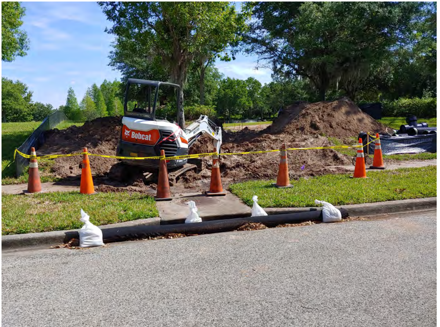
Installation of new drainage for playground west of Rose Cottage.
